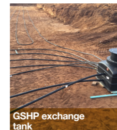
Excavation for GSHP
